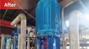
The original system has problems such as transmission gear box bearing oil leakage, high energy consumption etc. Permanent magnet direct drive retrofit completely eliminates the transmission gear box, lower down downtime and use a supporting frequency converter to control the motor operation, so as to achieve energy saving rate of 32.5%.
